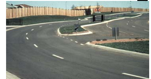
ABOVE FIG. 10-8: An example of poor transport / land use integration. The solid fences encourage greater vehicular speed, reduce visibility of the street by land uses and vice versa (diminishing safety), and often also encouraging vandalism.
