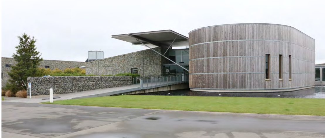
Selwyn District Council offices in Rolleston
